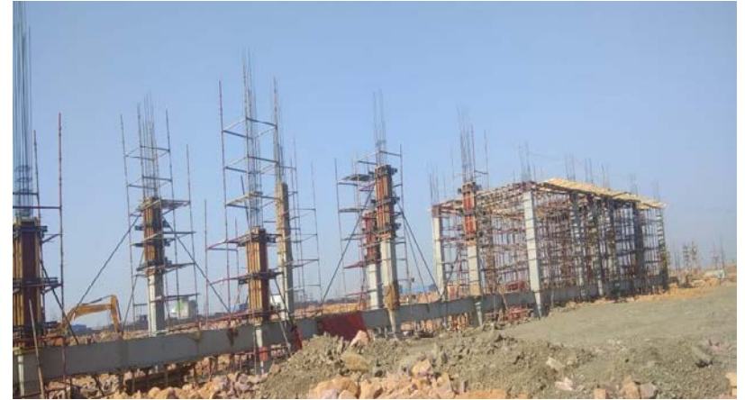
Engine line building
